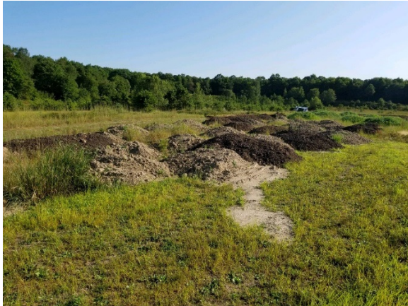
Stock piling Topsoil
